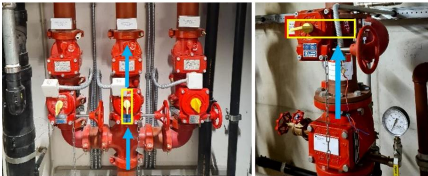
Figure B1.2 Left: Monitoring position (yellow button) in open position; valve is open. Right: monitoring position in closed position, valve is closed (Source: NIPV)
