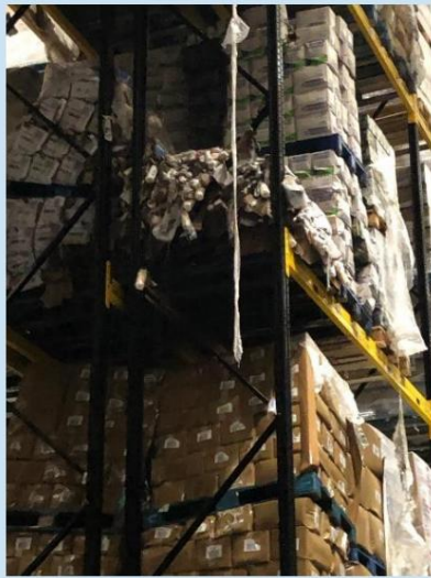
Figure 3.2 As a result of the fire, the wrapping film became loose (Source: TBO VGGM)
