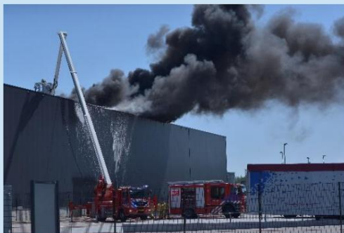
Figure 2.4 Roof on fire on a sprinklered warehouse (Source: TBO VRBZO)
