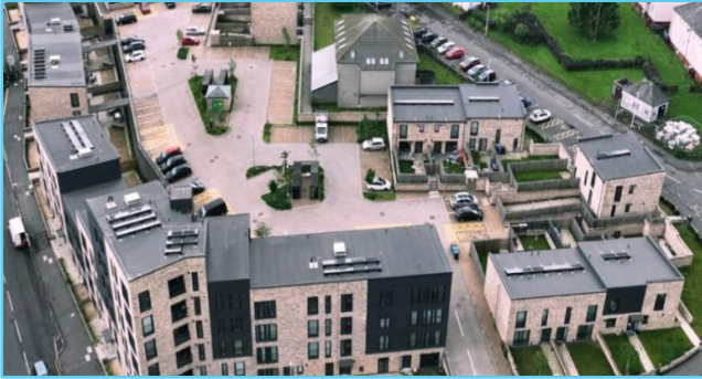
Credit image Discovery Fire Sprinklers Ltd
